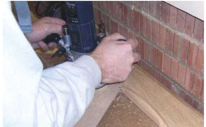
▲ Pic.7 Using a trammel to rout the curve on the middle rail (M)
